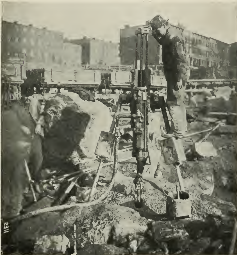
Drilling for P. R. R. Terminal Excavation.
